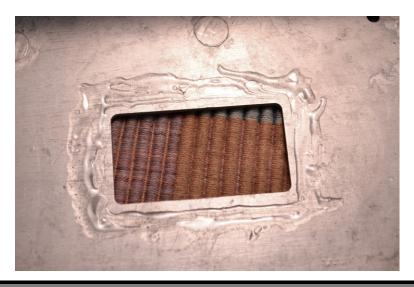
Carefully place the lens over the opening - **YOU ONLY GET ONE CHANCE** - so take your time and line it up before allowing it to contact the epoxy!!!
